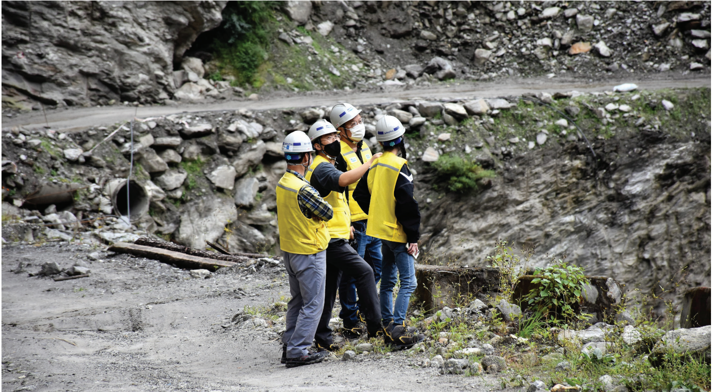
@Author/Photo/ Project EPC Contractors Inspecting the Diversion Dam Construction Site
