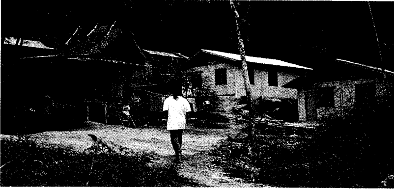
Plate 36. Cement houses for Muslim converts in Kampung Sungei Batu (Gombak, Selangor). As part of a positive discrimination programme, two recent converts in this village received the concrete houses on the right. Others, like the village headman seen here walking to his house, still live in traditional structures of bamboo, wood and atap. (CN-2000)
