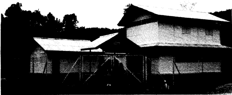
Plate 35. A community hall-cum-surau (Muslim prayer hall) in Kampung Sungai Serigala (Tanjung Malim, Perak). Despite the Orang Asli not asking for it, a programme to construct these structures in the early 1990s was implemented. The RM18 million (USD4.7 million) programme also included the training for 250 ‘welfare officers’ (by the Religious Affairs Department and the JHEOA) after which they were stationed in Orang Asli settlements. [CN-1992]
